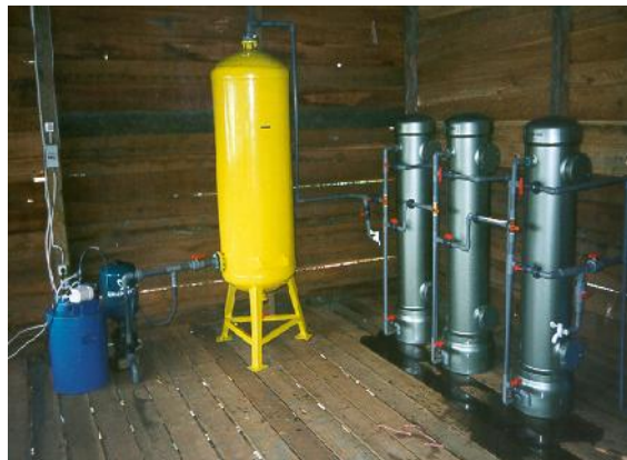
Gambar 19 : Sistem injeksi larutan kalium permanganat, filter pasir, filter mangan zeolit serta filter karbon aktif.
